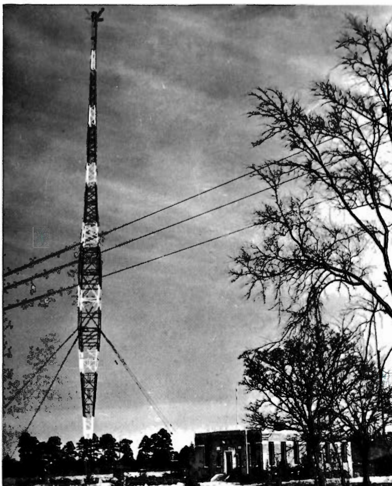
The New Vertical Radiator installed at Station WBT, Charlotte, N. C. This tower is 435 feet high
