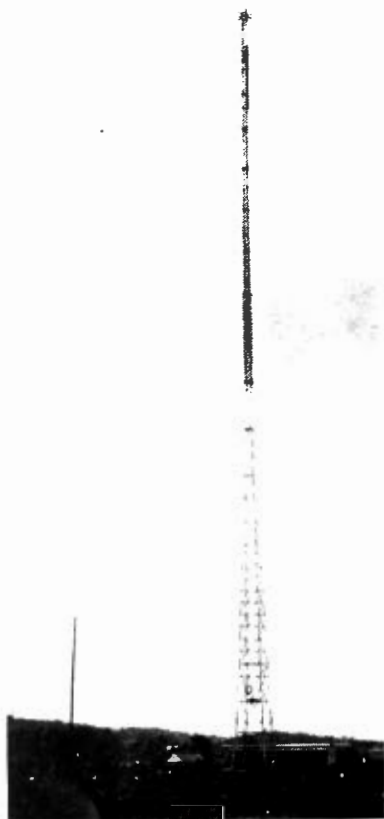
The new half-wave vertical radiator at WDOD
