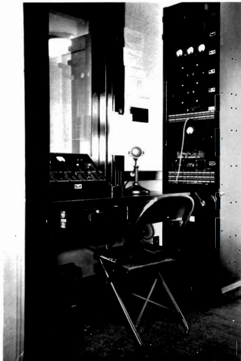
Corner of the control room at KSD showing RCA equipment in position
