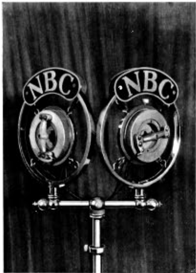
No. 6—The Hanson "Carbon Duo" microphone.
