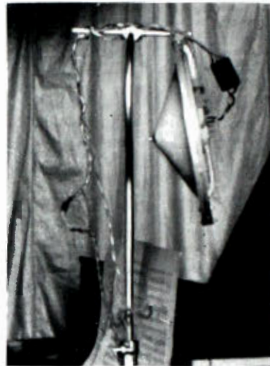
No. 2—The "dishpan" microphone—used at station WDY at Aldene, New Jersey, 1921-1922.
