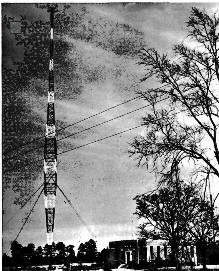
The New Vertical Radiator installed at Station WBT, Charlotte, N. C. This tower is 435 feet high
